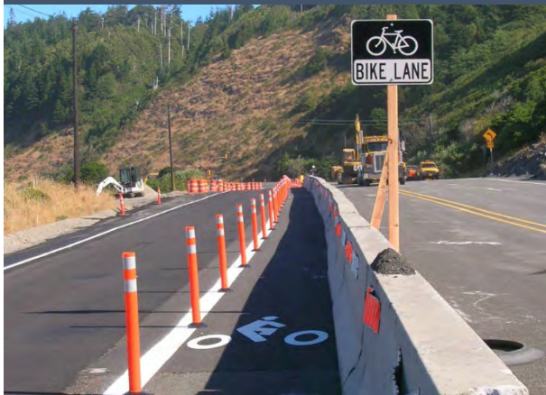
Work zone bike lane.
